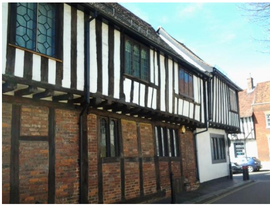
Number 37 showing different window styles and filled in cellar entrance
