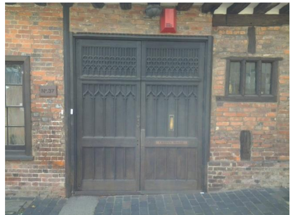
The 19C Gothic style carriageway entrance to number 37
