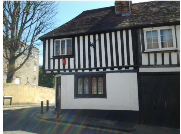
Refurnished ground floor of number 37, part of number 39 showing the carriage doors
