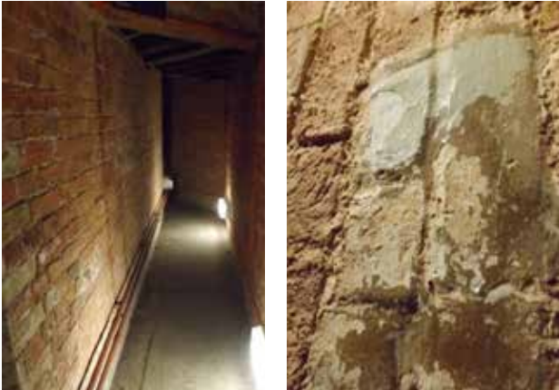
The sandblasted walls of the cells and corridor to cells
